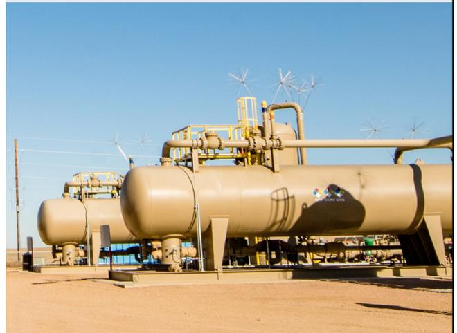
*Separators, like these in a natural gas gathering facility, can be inspected for gas leaks and checked for efficient operation.*
