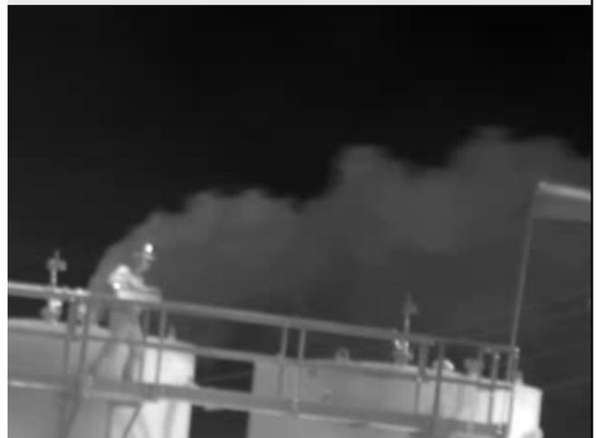
*Oil and gas industry worker on tank catwalk and inside gas leak from open thief hatch.*
